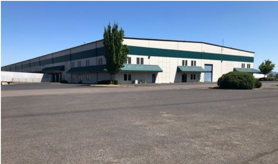
North West view
